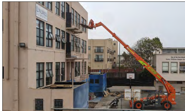
Retrofitting our high school building
